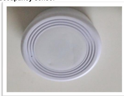
Picture 4: Telkonet ceiling mounted occupancy sensor
